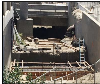
Elevator foundation on Metro R/W requires only forming and concrete pour
