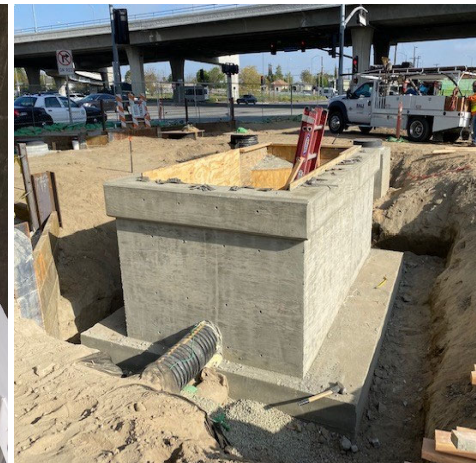
Formed & poured North Drainage System
