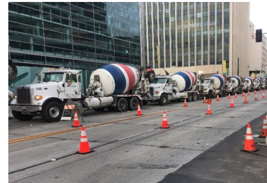
First Concrete Placement for Wilshire/Rodeo Station Invert
