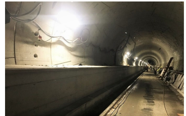
Reach 1 Tunnel Invert & Walkway Concrete Placement
