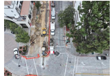
Holly and Arroyo Westbound Station Construction
