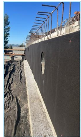
Drain board on Van Nuys Abutment 5 Back Wall
