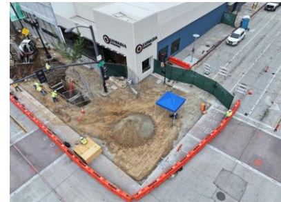
Colorado and Lake Westbound Station Construction
