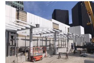
Century City Station Canopy Installation
