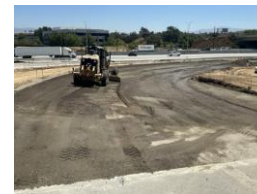
Aggregate Base Valencia SB Onramp
