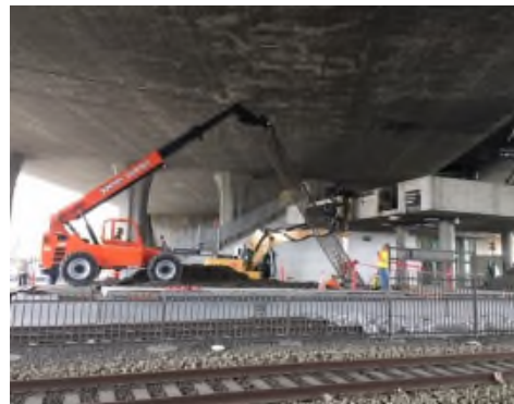
Demolition of Rail Platform and Mezzanine
