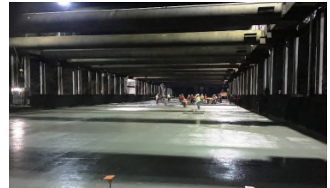
Placement of Mud Mat at Wilshire/Fairfax Station
