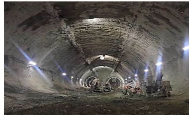
SEM Cavern excavation completed
