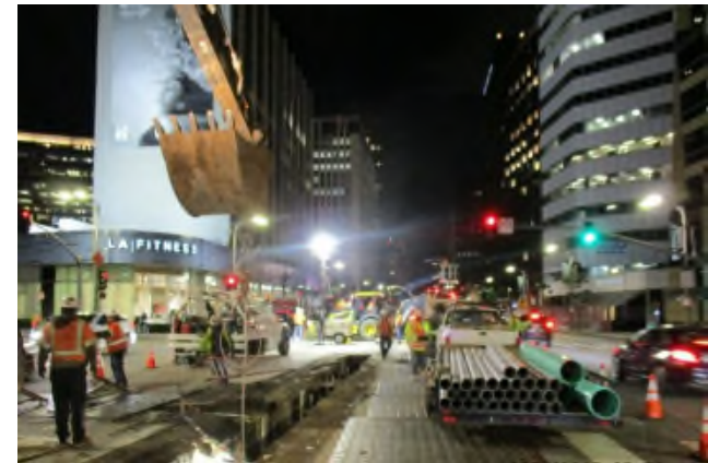
LADWP Water Pipe, Valve and T-Section Installation
