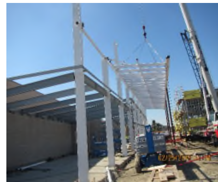
Structural Steel Installation for Mobility Hub
