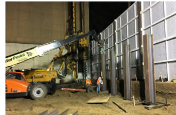
Muck Bin Pile Installation
