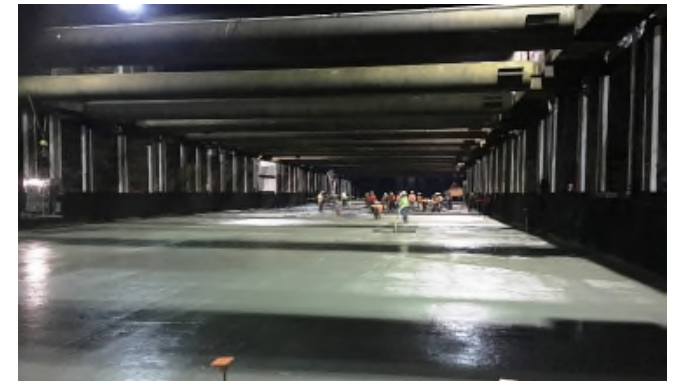
Placement of Mud Mat at Wilshire/Fairfax Station
