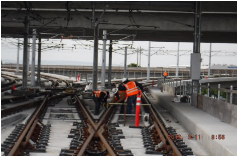
Contractor aligning trackwork at south end Green Line tie-in
