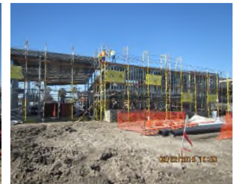
Framing for Customer Service Building
