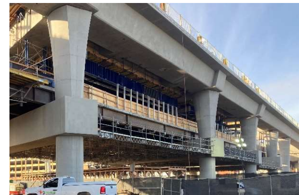
LAWA Station work in progress
