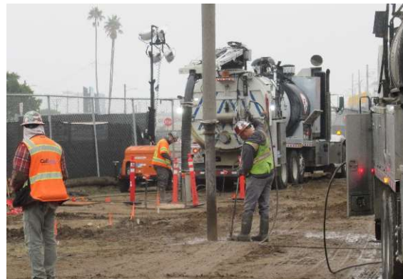
Shoring installation for Stormwater System
