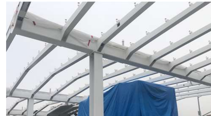
Little Tokyo/Arts District Station Canopy Installation
