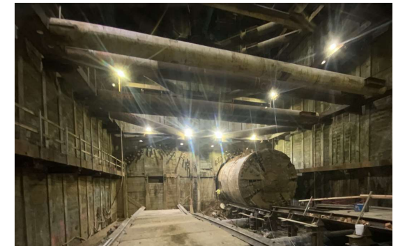
Harriet Breakthrough at Wilshire/Rodeo Station
