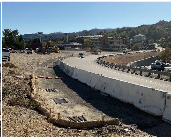
Placement of temporary work zone speed radar and stormwater pollution prevention materials
