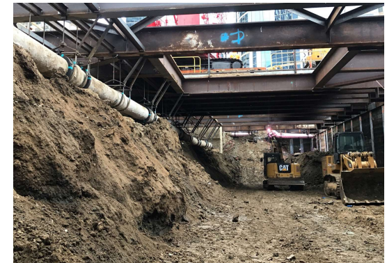
Constellation Station Entrance Excavation
