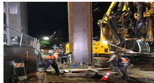
SOE Pile Installation Along North Side Wilshire Blvd.
