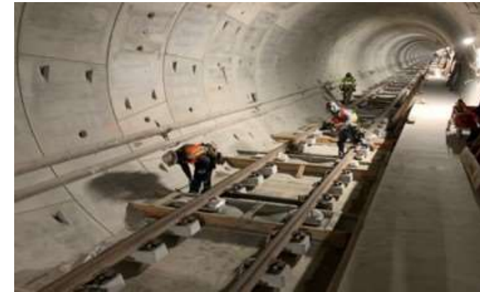
Reach 1 North Tunnel Trackwork Installation
