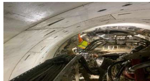
Ring Installation in the BL Tunnel
