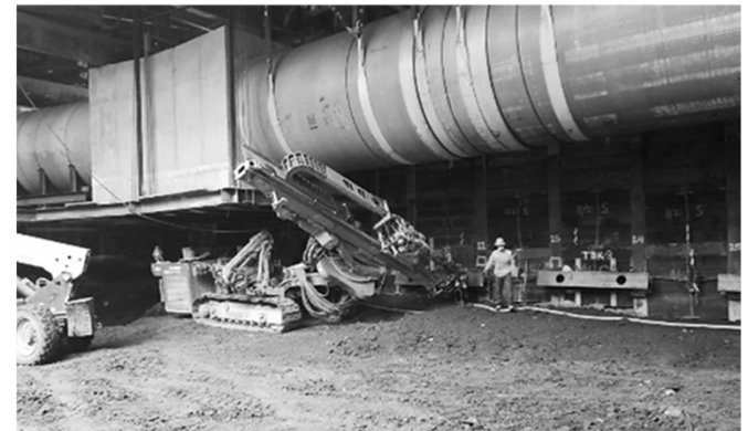
Tieback installation at Historic Broadway Station
