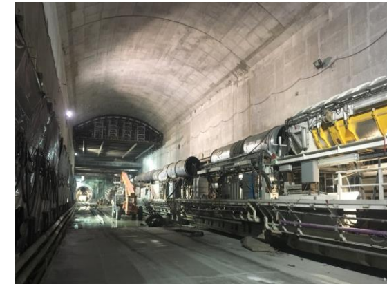
TBM Gantries at Wilshire/La Cienega Station
