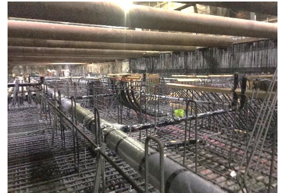
Rebar work for Wilshire/Rodeo Station Invert
