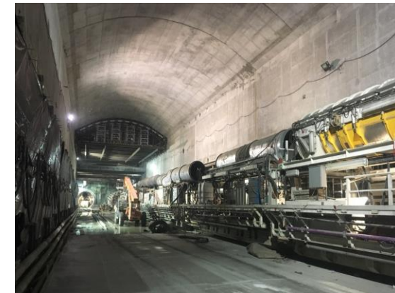
TBM Gantries at Wilshire/La Cienega Station
