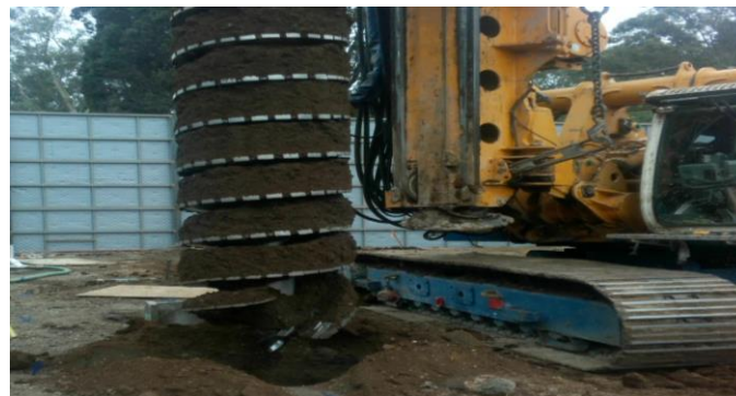
Drilling for Support of Excavation Soldier Pile Installation at Westwood/VA Station
