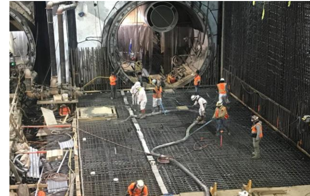
Wilshire/La Brea West Hammerhead Concrete Placement
