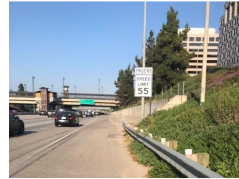
Newly Installed Speed Limit Sign
