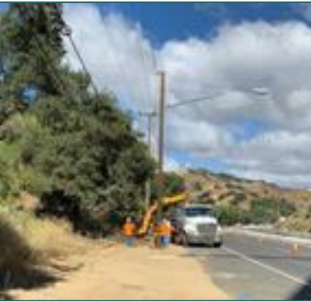
Old Road-SCE Power & AT&T Relocation
