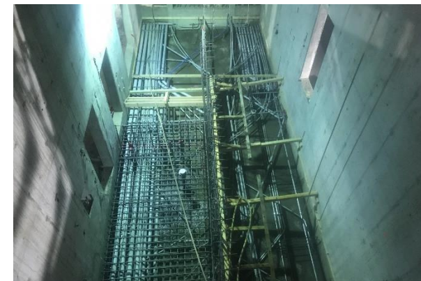
Track Level Conduit Installation at Wilshire/La Brea
