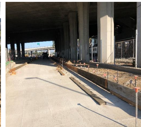
Hardscape Work @ Central Plaza
