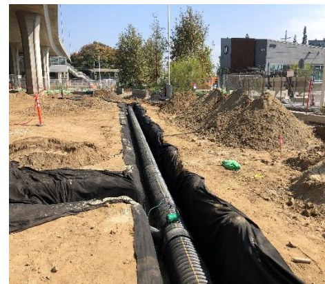
Utility Work @ Package B
