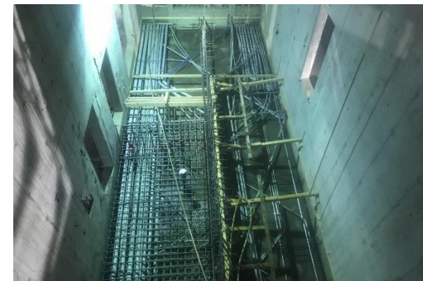
Track Level Conduit Installation at Wilshire/La Brea
