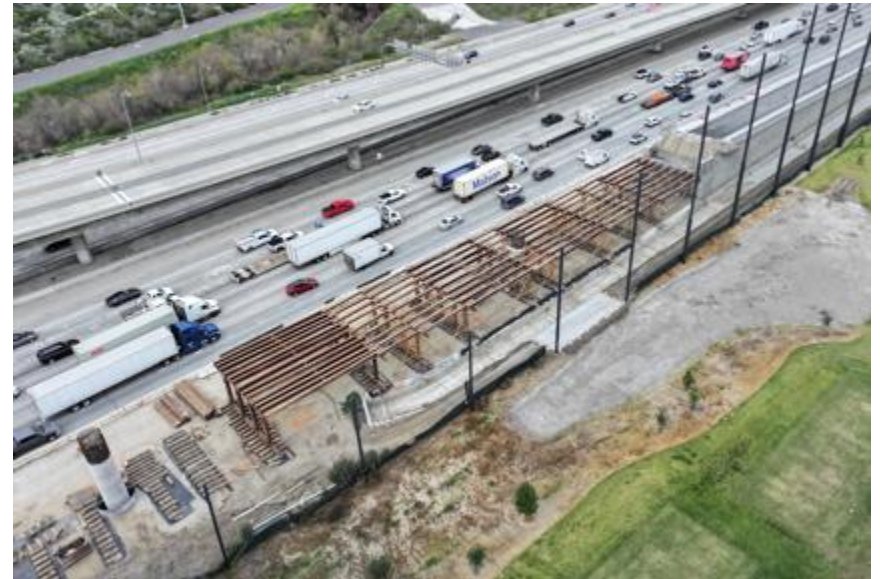
Erection of falsework for EB60-Grand Ave/N57 Separation
