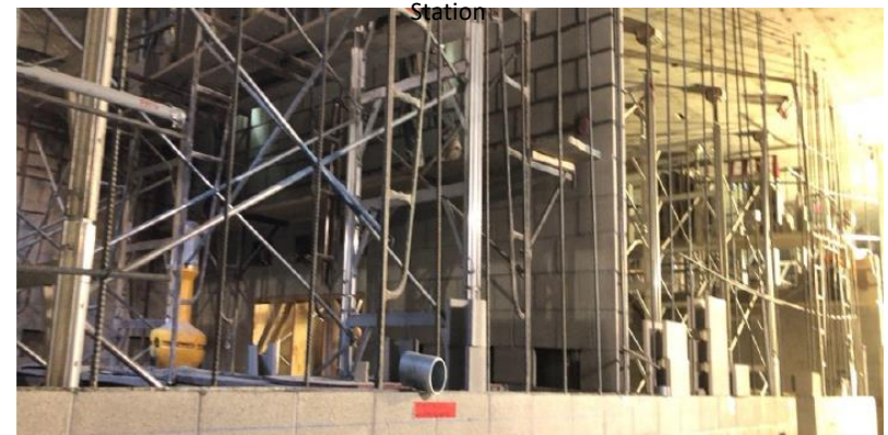
Conduit installation at CMU walls
