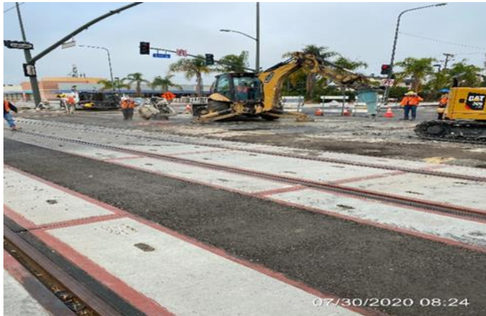
Excavating/removing section of pavement for restoration on southbound Crenshaw Blvd and 54th St.
