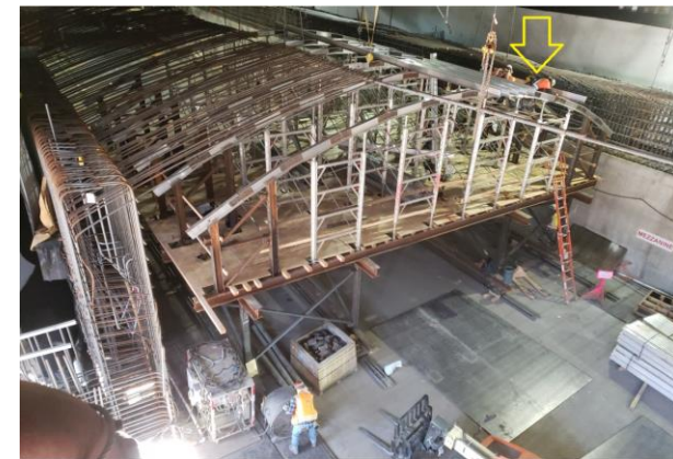
Installing Roof Falsework at Wilshire/Fairfax Station
