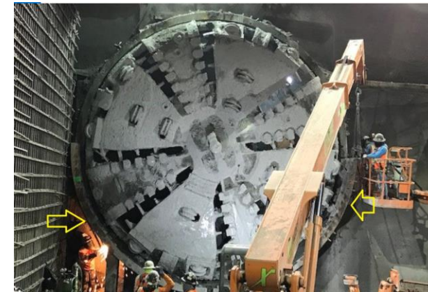
Purple TBM Arrival of Wilshire/La Cienega Station
