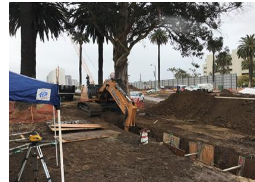
Storm Drain Relocation West of Bonsall Westwood/VA Station
