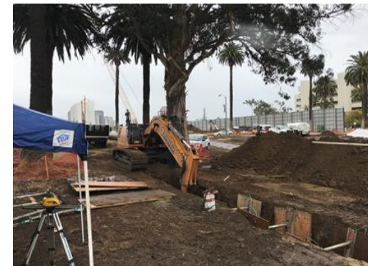
Storm Drain Relocation West of Bonsall Westwood/VA Station
