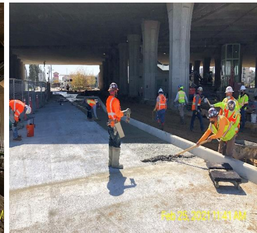
Phase 3 Curb and Bus Lane completed
