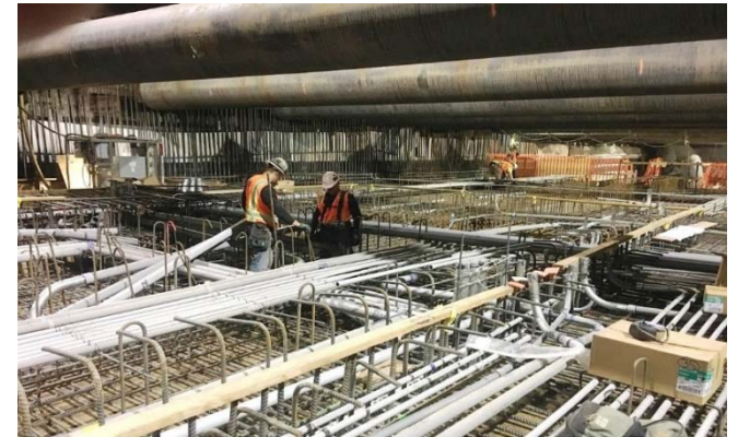
Installation of Conduit at Wilshire/La Brea Station
