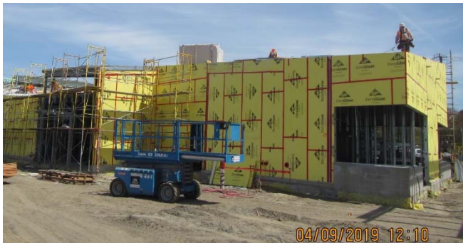
Exterior sheathing at Customer Service Building
