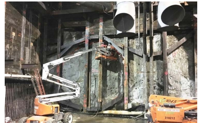
Reach 2 Tunnel Ring Installation at Wilshire/La Brea Station
