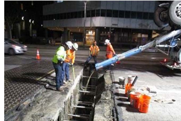
Slurry Backfilling Laterals on Wilshire Blvd.
