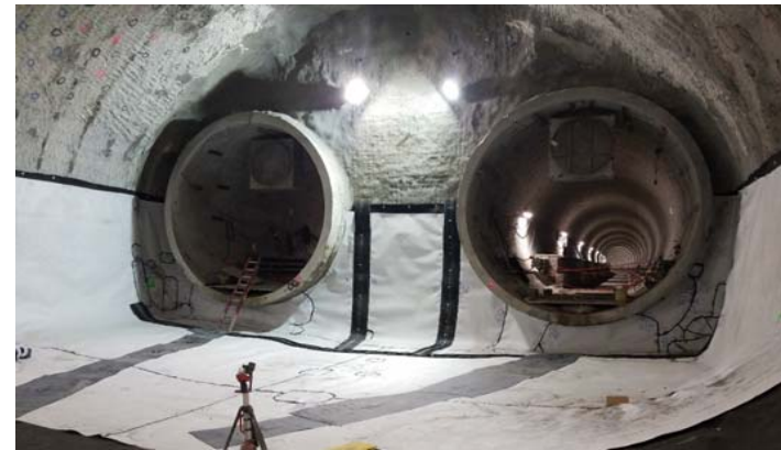
HDPE installation at SEM Cavern headwall
