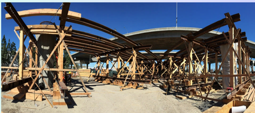
Crenshaw tie-in with Green line falsework construction
