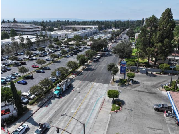
Potholing Early Works Package in Pasadena
