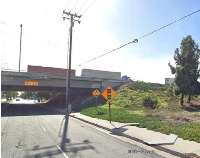
Utilities Relocation at Norwalk Blvd. (North SR-91)
