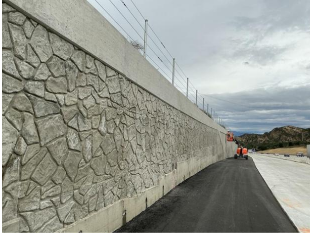
Roadway Excavation Southbound Hasley to Parker
