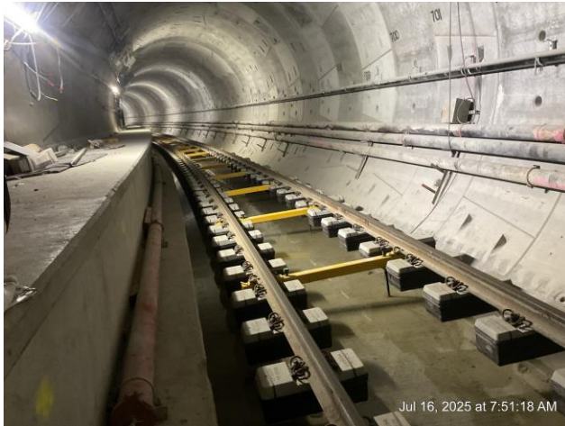
BR Tunnel Reach 5 Track Installation
