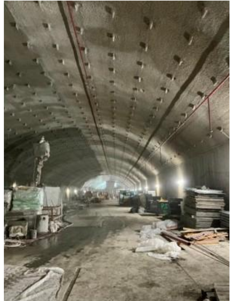
Westwood/VA Hospital Station Arched Roof
