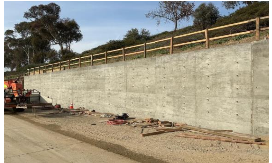
Stripping of forms from retaining wall
