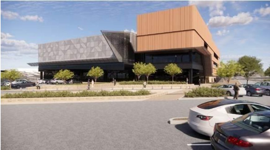
Building Exterior - West View
