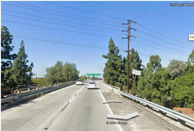
WB 91 to 605 Connector - Utilities Relocation at Studebaker
