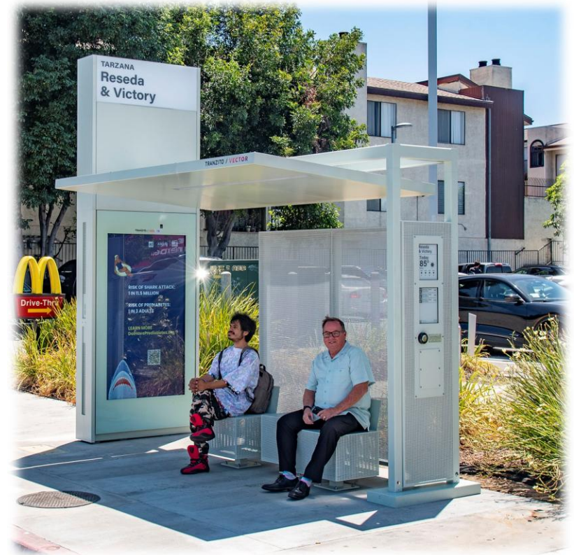
Bus shelter installed at Reseda and Victory
