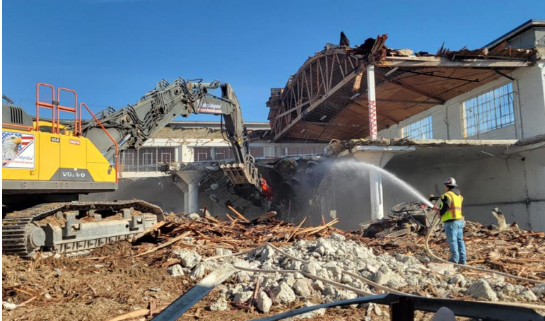
Life Storage building demolition (March 2025)
