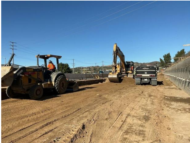
Calgrove Off-Ramp Gore Area Concrete Preparation
