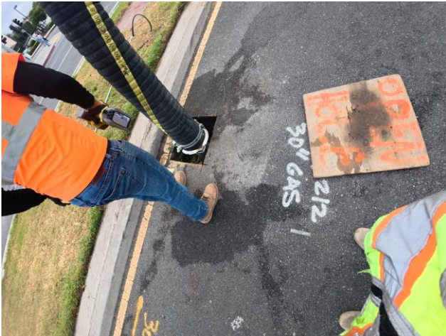
Potholing Early Works Package in Glendale
