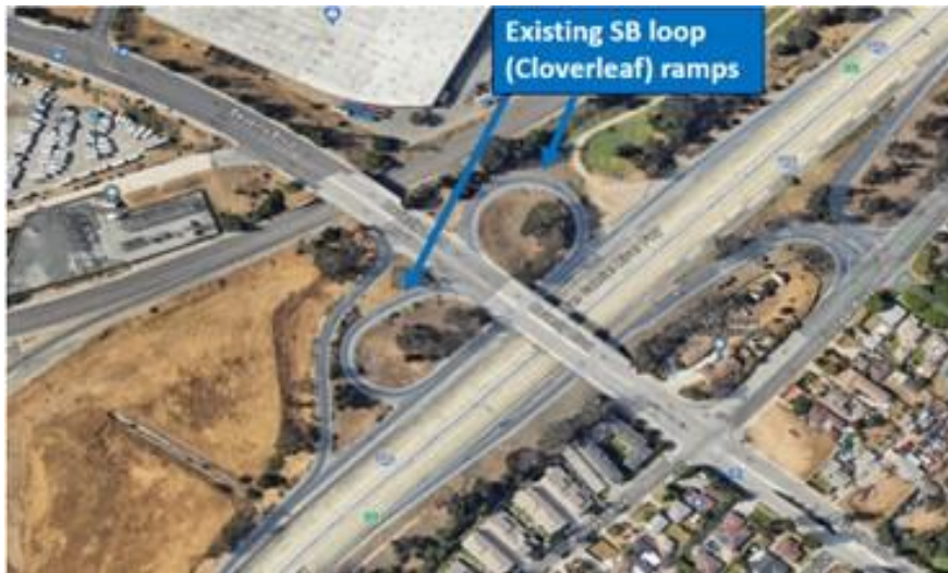
Aerial View of Existing Beverly Blvd.
