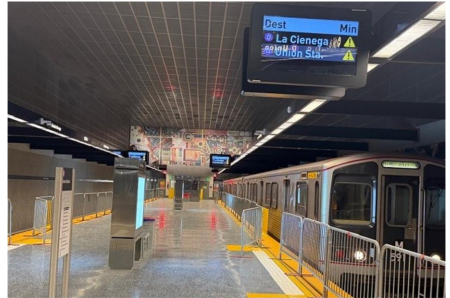
Test Train at Wilshire/La Cienega Station Platform
