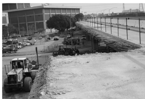
Edge of Deck Removal
