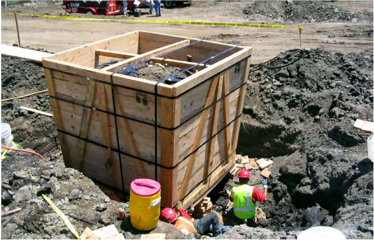
Fig 10: Tunnel under the tree box
