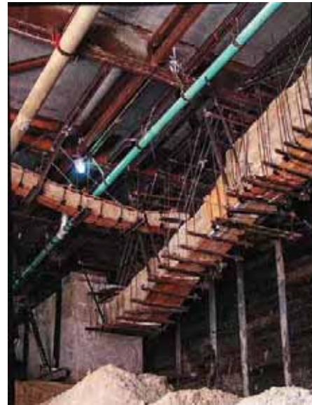
Figure 3-18: Utilities Hung from Deck Beams (Close Up)
