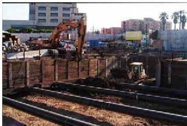
Figure 4-5: Open Cut Excavation of Side Access Shaft
