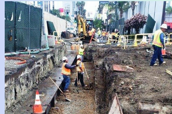
Wilshire/La Brea Station – Preparation for Deck Beams
