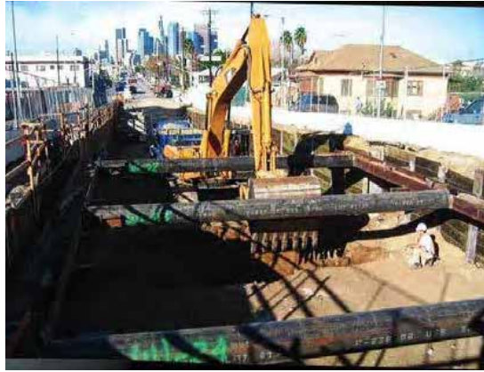
Figure 4-12: Hydraulic Excavator between Struts
