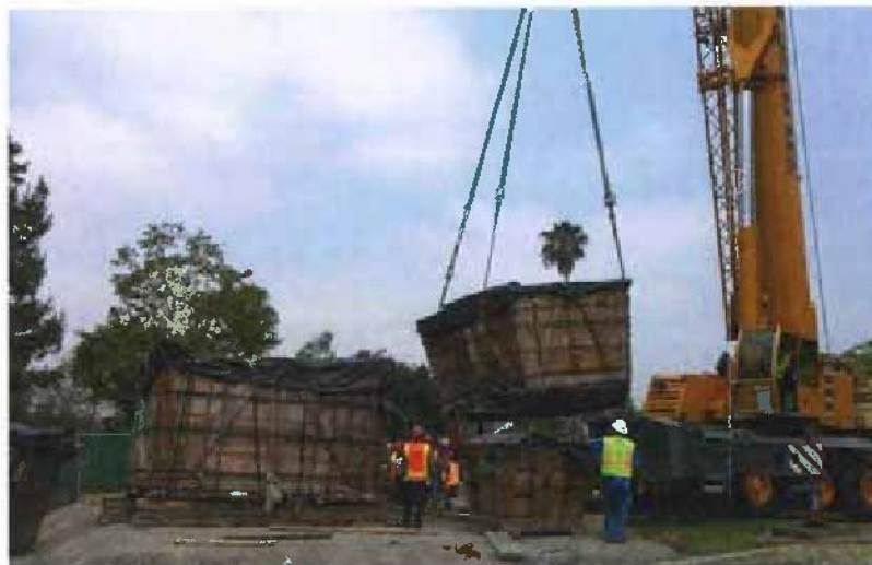
Figs 11, 12 & 13: Relocating the tree boxes by crane and truck
