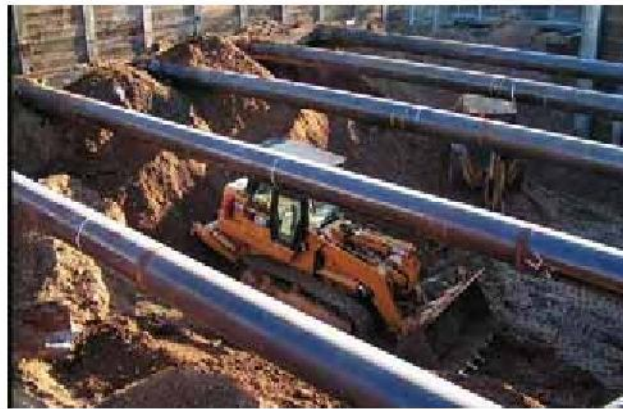
Figure 4-13: Track Loader beneath Struts
