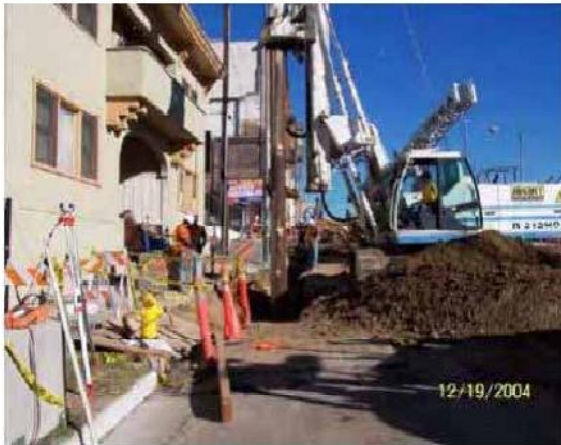
Figure 3-7: Pre-augering for Soldier Pile
