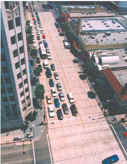
Figure 3-1: Roadway Operations Restored on Temporary Decking System
