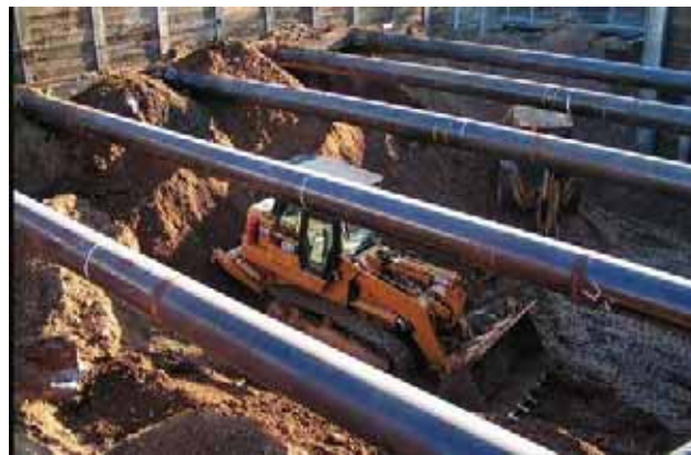
Figure 4-13: Track Loader beneath Struts
