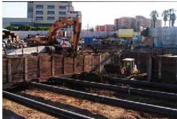
Figure 4-5: Open Cut Excavation of Side Access Shaft
