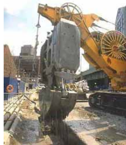
Figure 3-15: Clamshell Digger for Slurry Wall Construction
