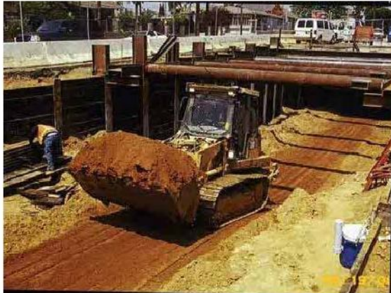
Figure 4-13: Track Loader beneath Struts
