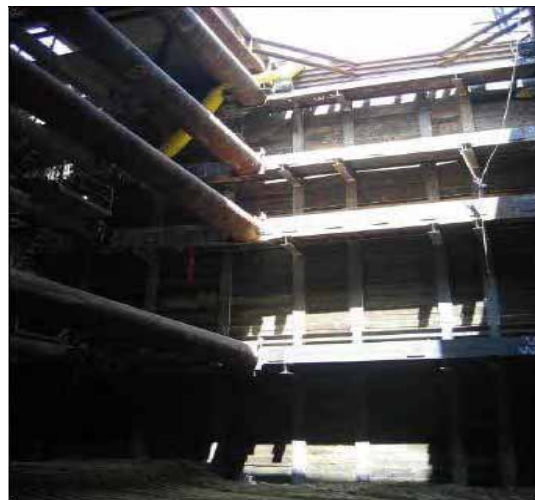
Figure 3-9: Soldier Pile and Lagging
