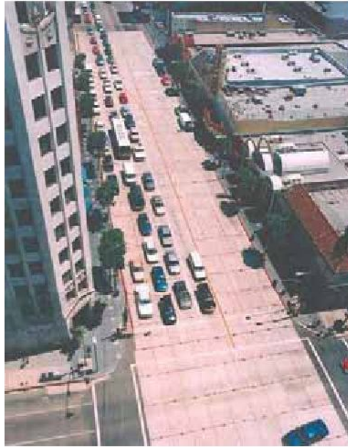
Figure 3-6: Roadway Operations Restored on Temporary Decking System
