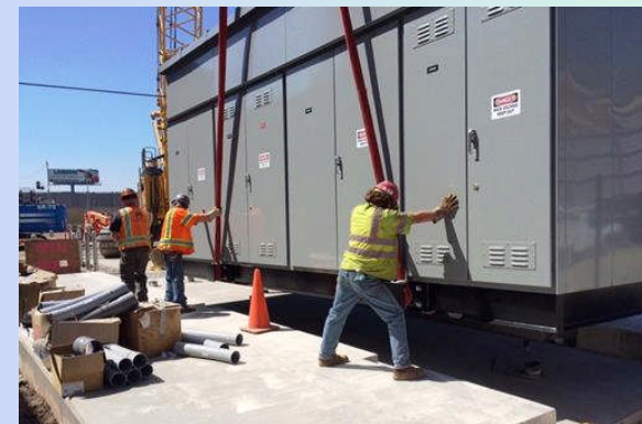
Electrical Metering Switchgear for Tunnel Operations
