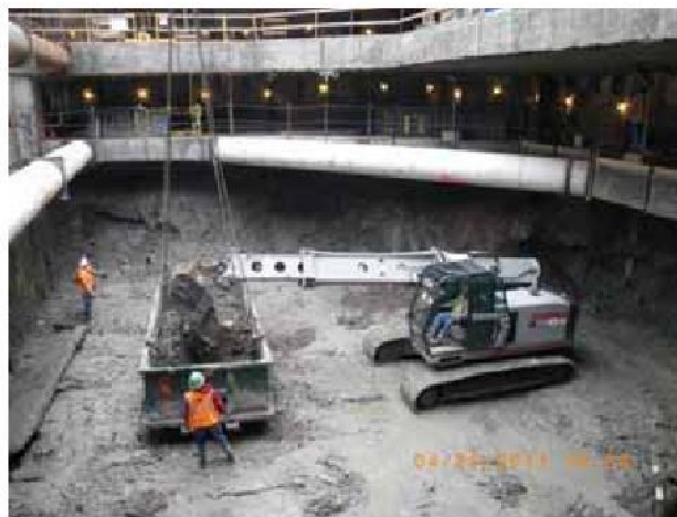
Figure 4-6: Gradall Excavator - East Side Access Project NYC
