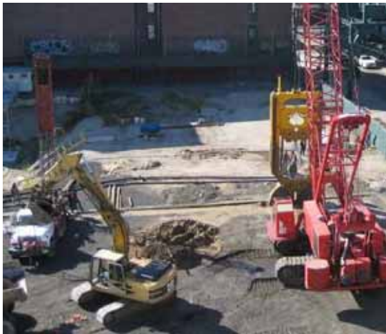
Figure 3-14: Slurry Wall Construction Equipment
