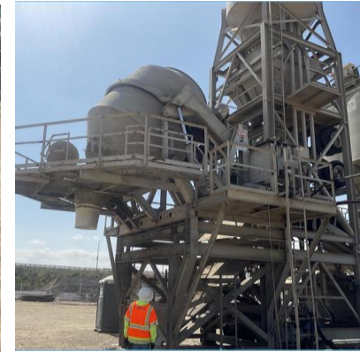
On-site concrete batch plant
