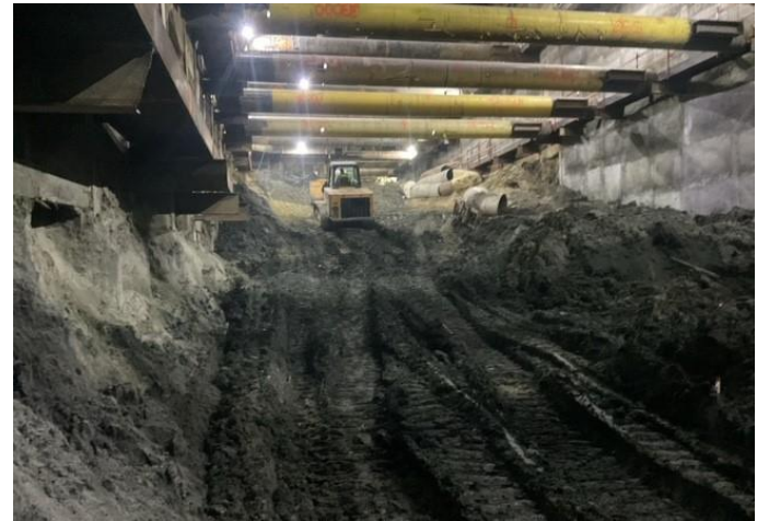
Century City Constellation Station - Excavation Progress
