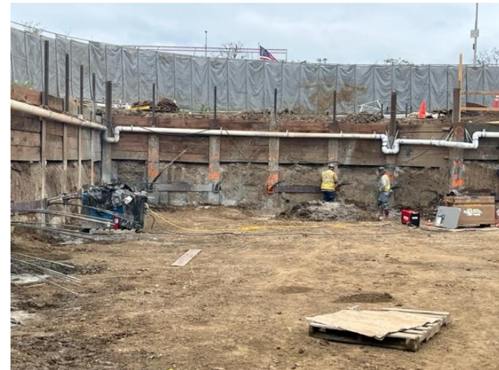
Westwood/VA Station: Tiebacks Installation– North & West Walls
