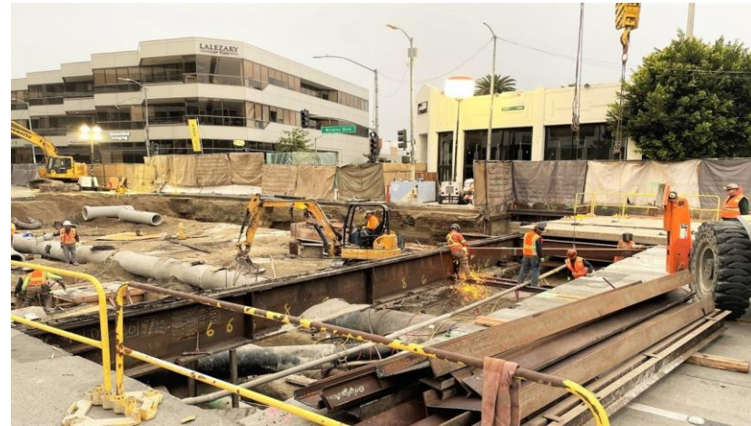
Wilshire/La Cienega Deck Removal/Street Restoration
