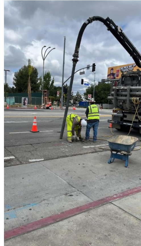
Potholing at Van Nuys Blvd
