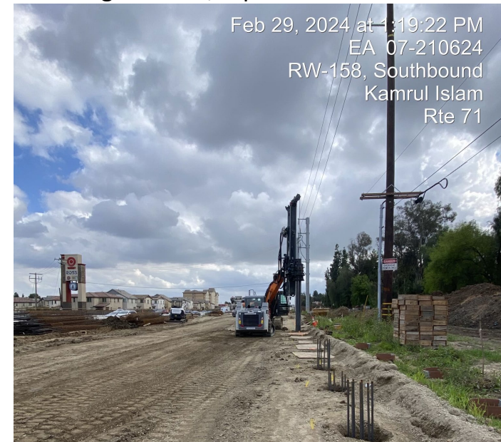
SR-71 SB, SW158 CIDH pile construction.
