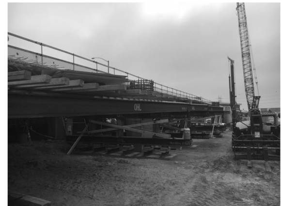
False work on south side
