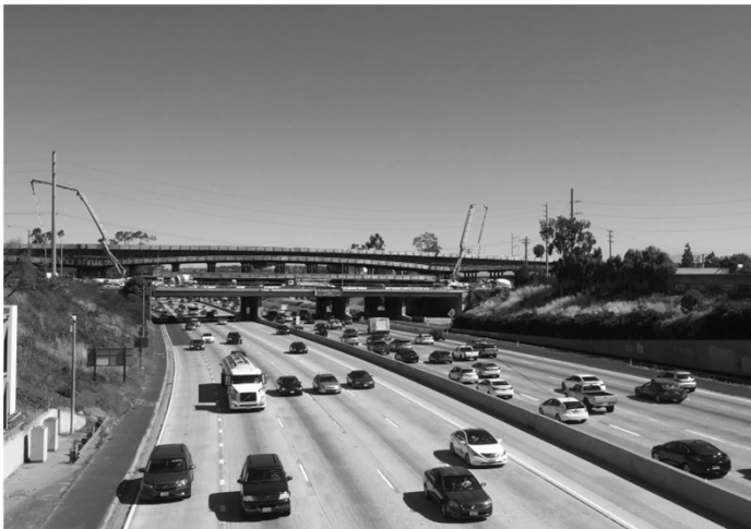
Completed deck concrete placement for I-405 bridge structure.
