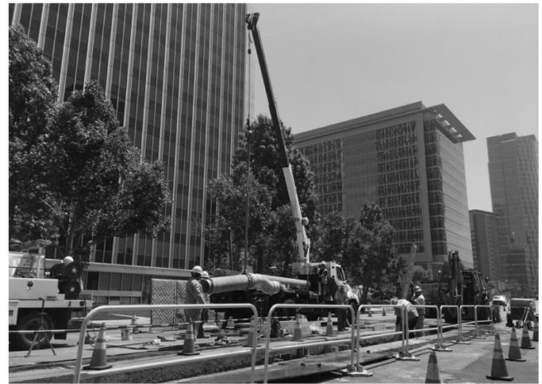
LADWP water relocation work in Century City
