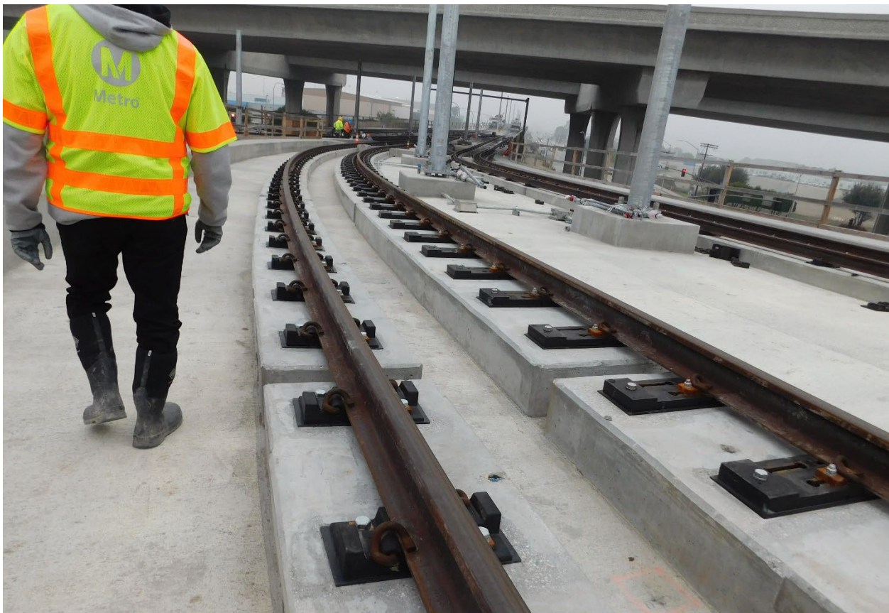
Crenshaw project – K Line - Elevated concrete fixed rail above Imperial Highway and below 105 Freeway
