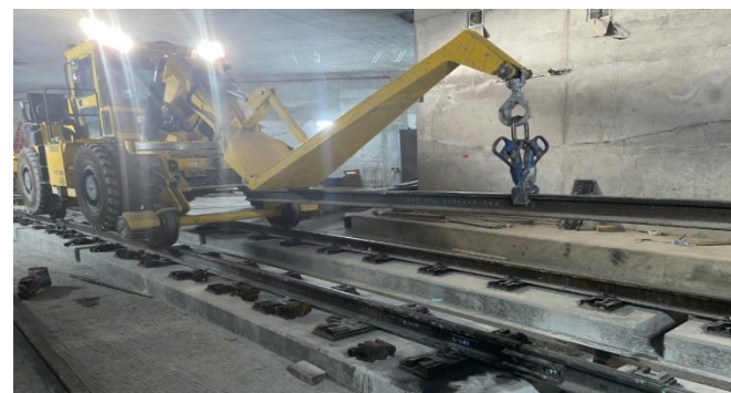
1st Street Leg Plug Rail Installation
