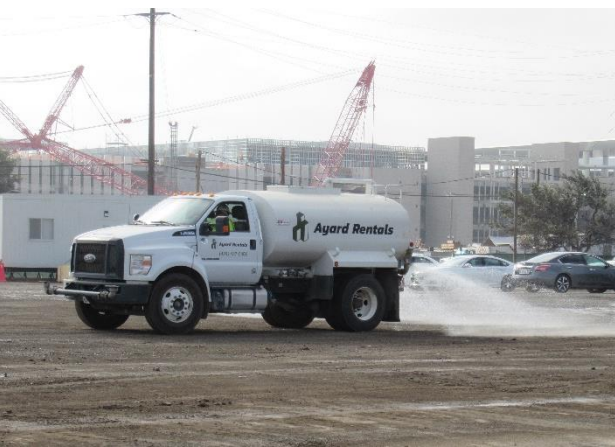
Grading Work continues
