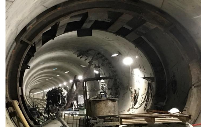
Reach 2 Cross-Passage Excavation Preparation
