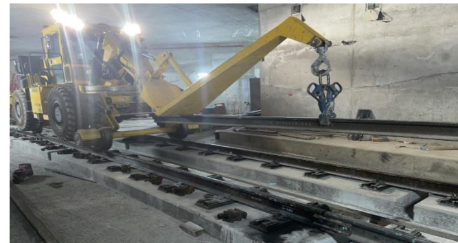
1 st Street Leg Plug Rail Installation
