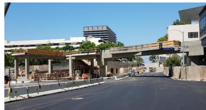
Asphalt pavement complete along Hope Street
