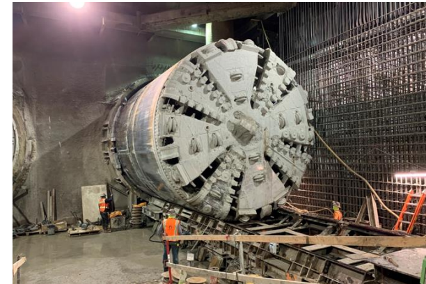
Red TBM Arrival of Wilshire/La Cienega Station
