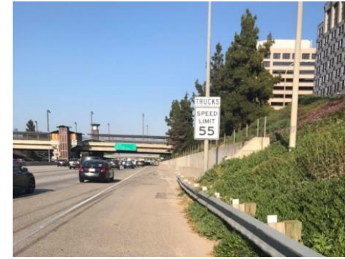
Newly Installed Speed Limit Sign
