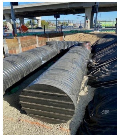
Installed cistern for North GSRD
