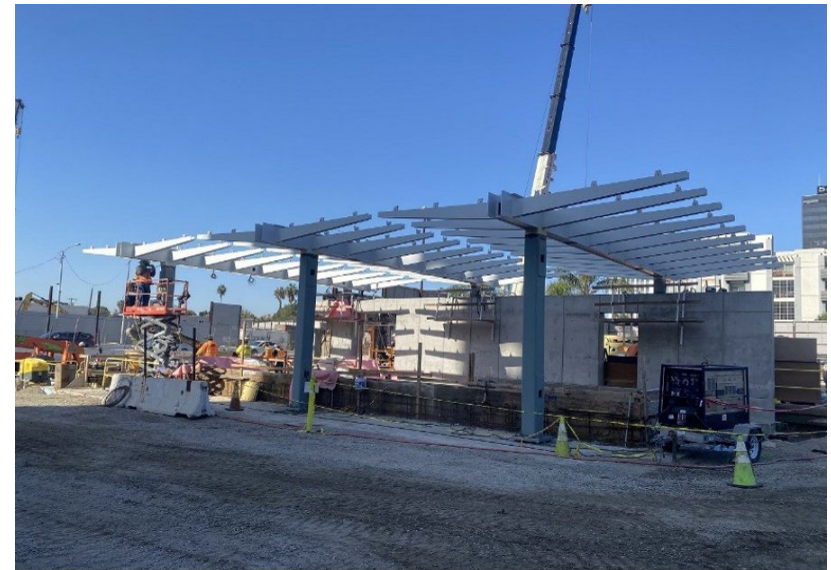
Wilshire/La Brea Station Canopy
