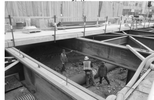
Hanging in place utilities under street decking at Wilshire/La Brea Station
