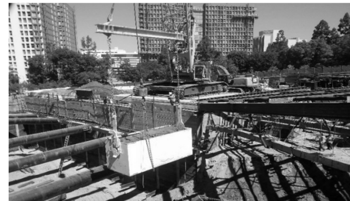
Muck Removal at 2nd/Hope Station
