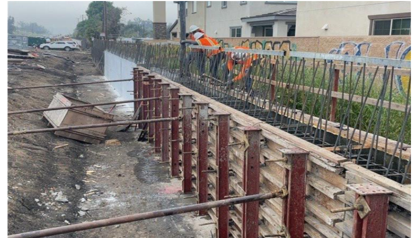
Retaining wall 161 construction
