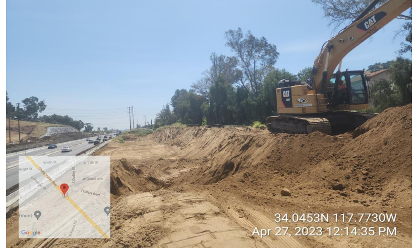
Excavation along southbound roadway
