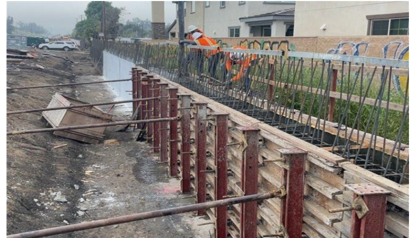
Retaining wall 161 construction
