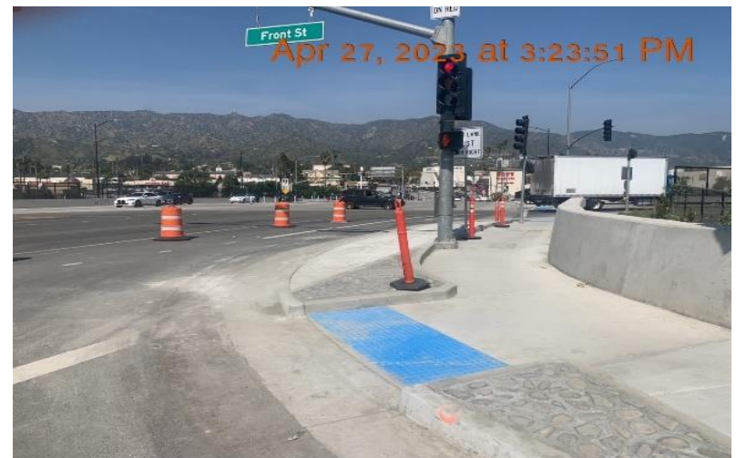
Bike lane improvement at Burbank Blvd overcrossing
