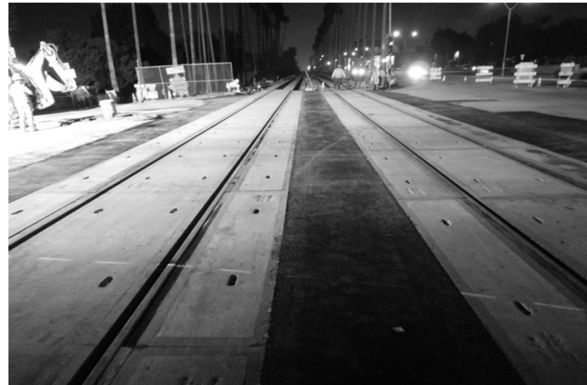
Completed first grade crossing at Centinela Avenue
