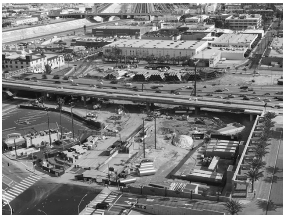
Aerial view of site
