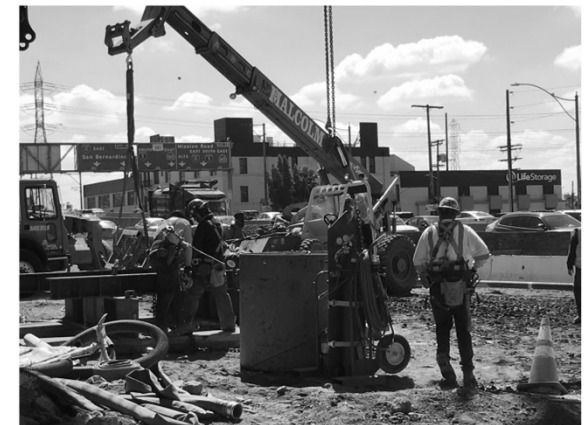
Setting and Pouring Bent 4
