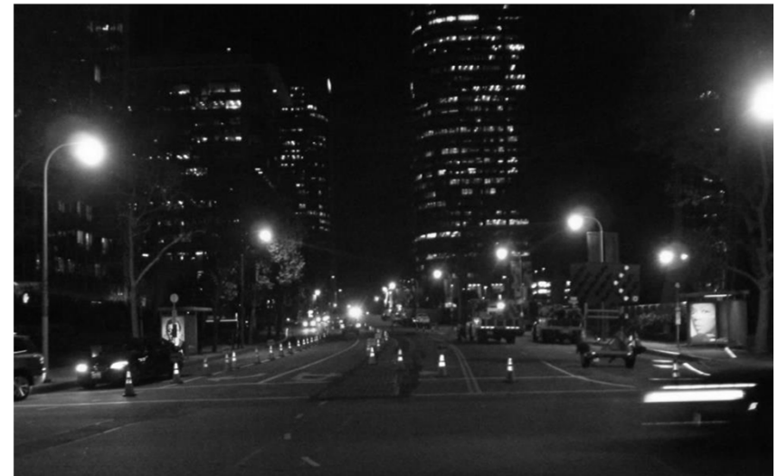
Telecom Joint Trench Construction along Constellation Boulevard
