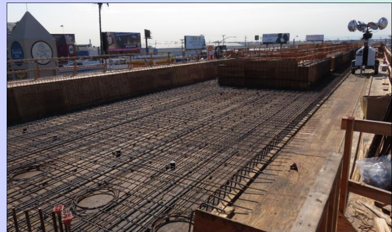
AVIATION/CENTURY BRIDGE – Rebar Installation
