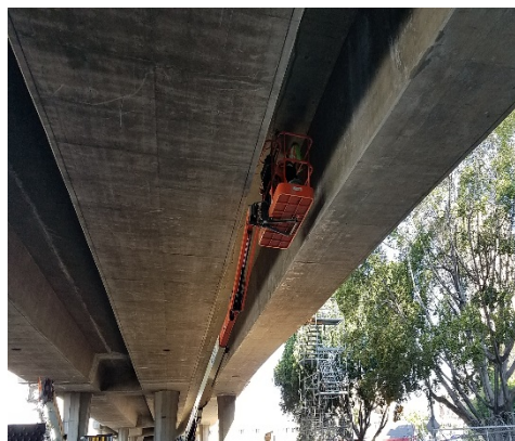
Concrete Finish Work
