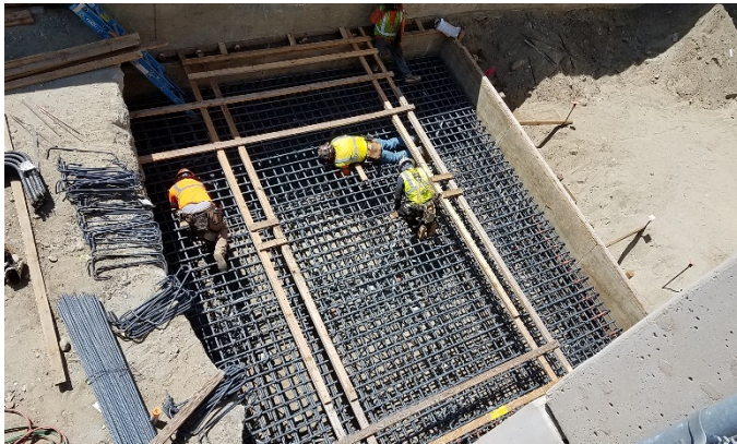
Elevator Footing Forming/Rebar
