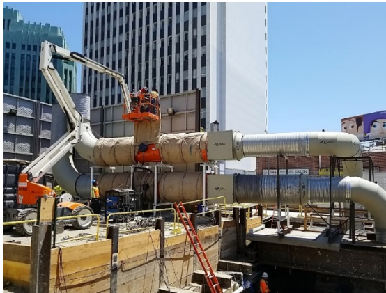
Wilshire/Western Retrieval Shaft
