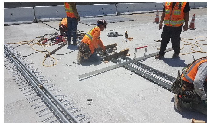
Joint Seal Assembly Install
