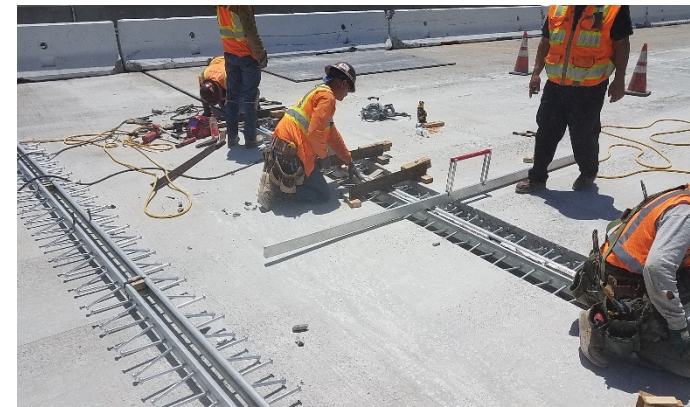
Joint Seal Assembly Install
