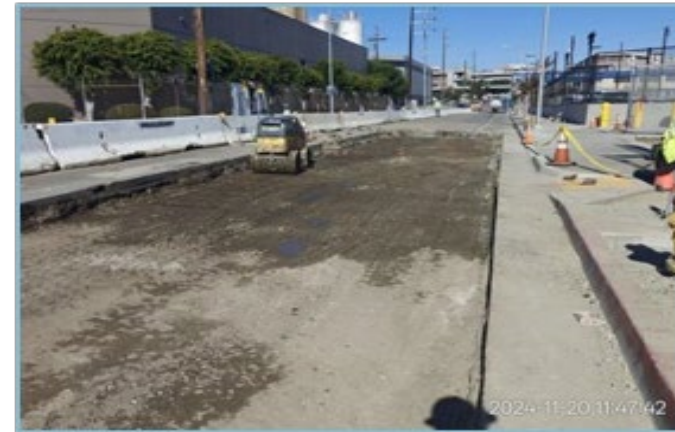
Center Street Reconstruction
