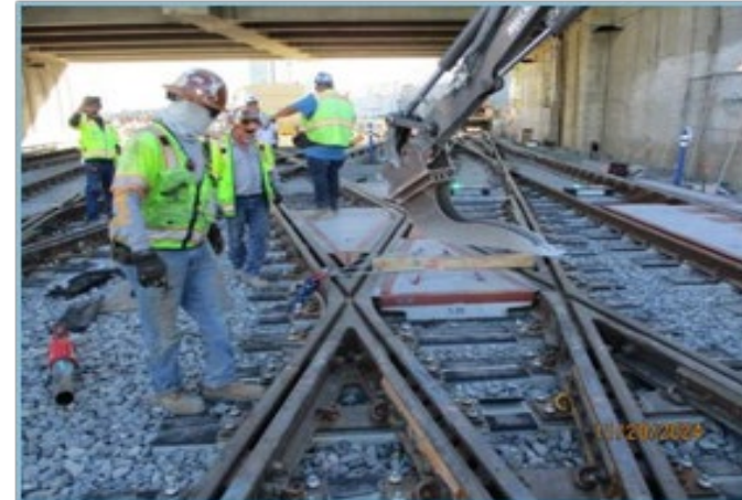
Crossing Panel Installation
