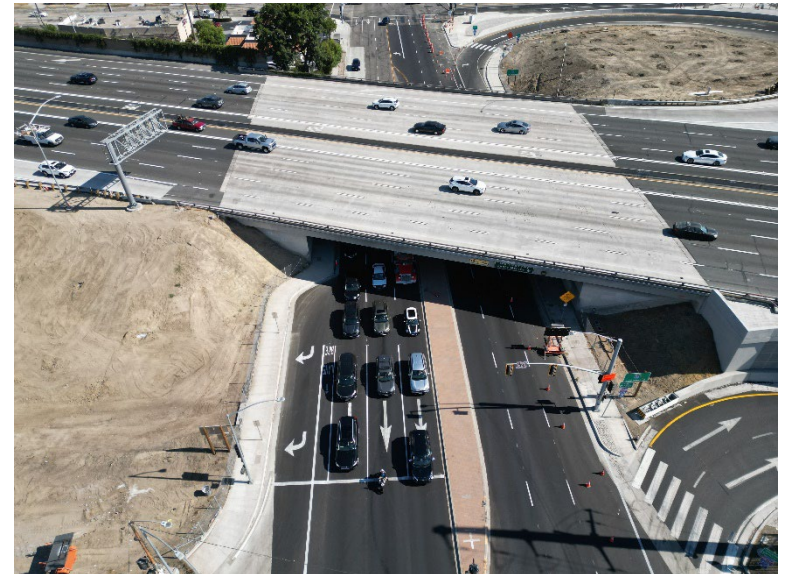
South side of Crenshaw Blvd UC (Looking North) showing Crenshaw Blvd improvements/auxiliary lane for realigned SB on ramp and new NB Crenshaw Blvd to SB 405 on ramp
