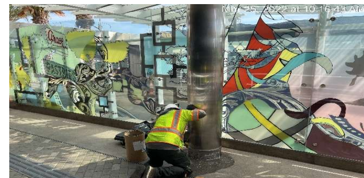
Hyde Park Station – Applying anti-graffiti shield
