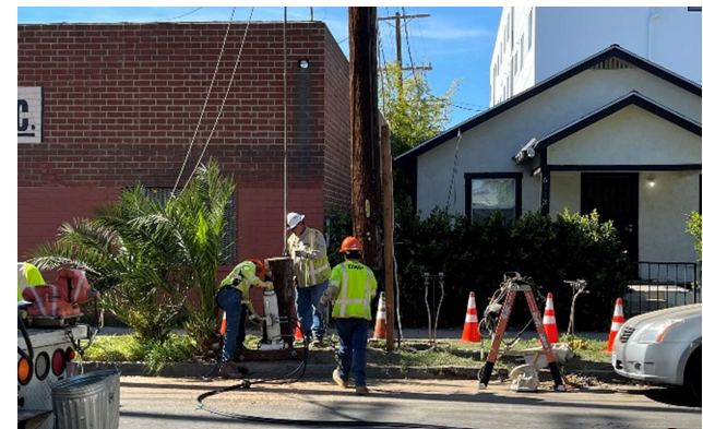
DWP Vesper Advanced Utility Relocation
