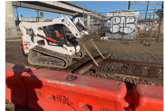
Removing ties for load out
