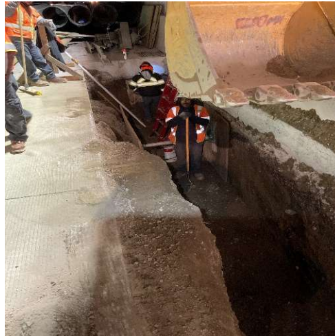
Drainage excavation on SB I-5 median DS# 159
