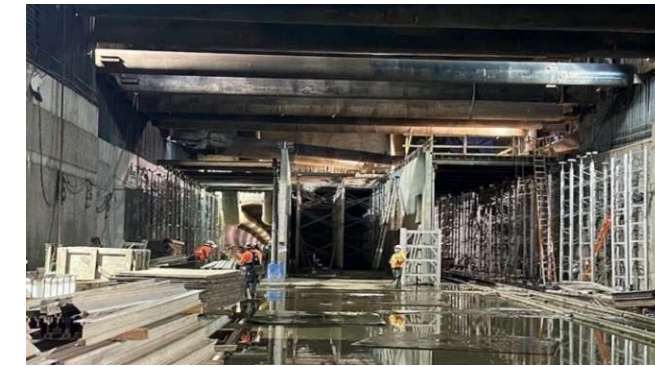
Shoring Tower Installation at Wilshire/La Cienega Station
