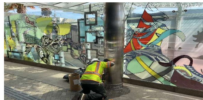
Hyde Park Station – Applying anti-graffiti shield
