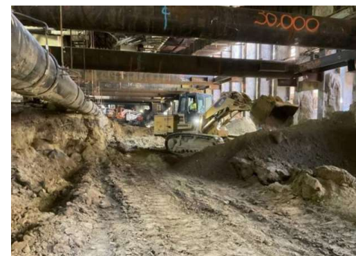
Century City Constellation Station Box Excavation
