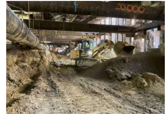
Century City Constellation Station Box Excavation
