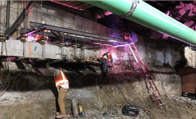
Utility support installation for DWP Power and Storm Drain Box on Flower St
