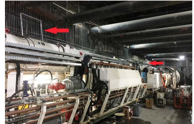
TBM Assembly at Wilshire/La Brea Station
