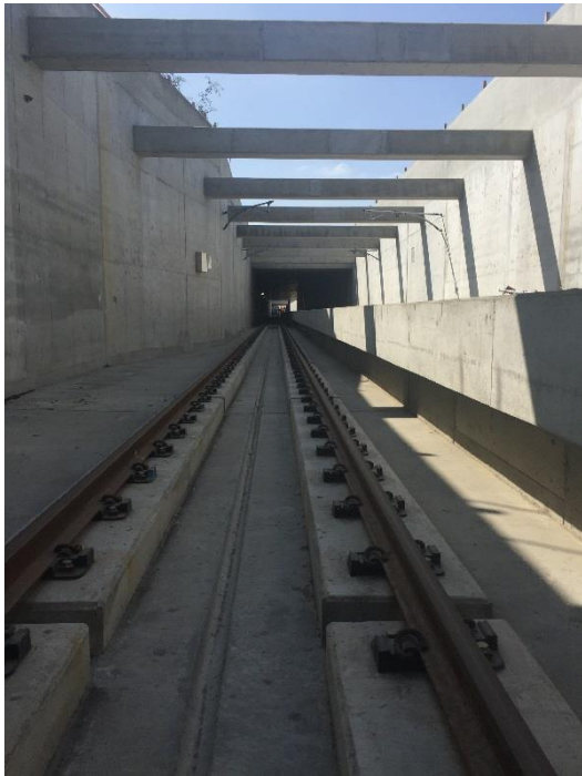
UG-1 - Tunnel section without the cover
