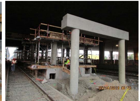
Pile and Beam work at Blue Line Platform/Mezzanine
