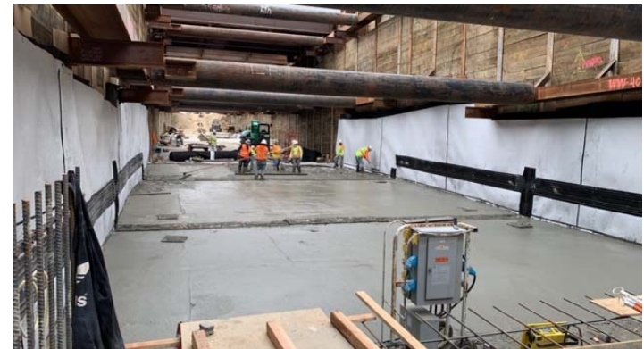
Protection slab placement at 1st Street Leg
