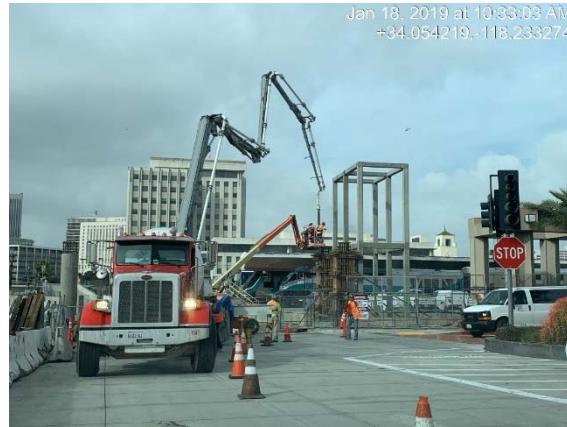
Pouring columns for the elevator structure
