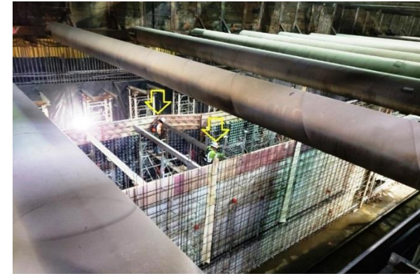
Wilshire/Fairfax Station Interior Wall Formwork
