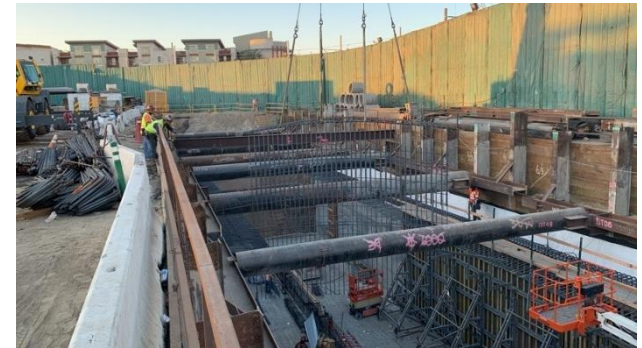
Exterior wall segment installation at Alameda Leg
