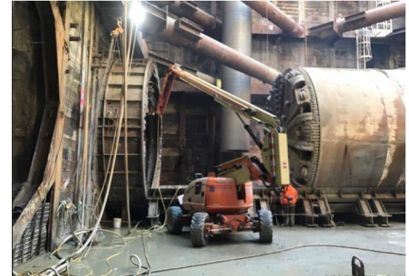
BL TBM “Ruth” at Tunnel Access Shaft
