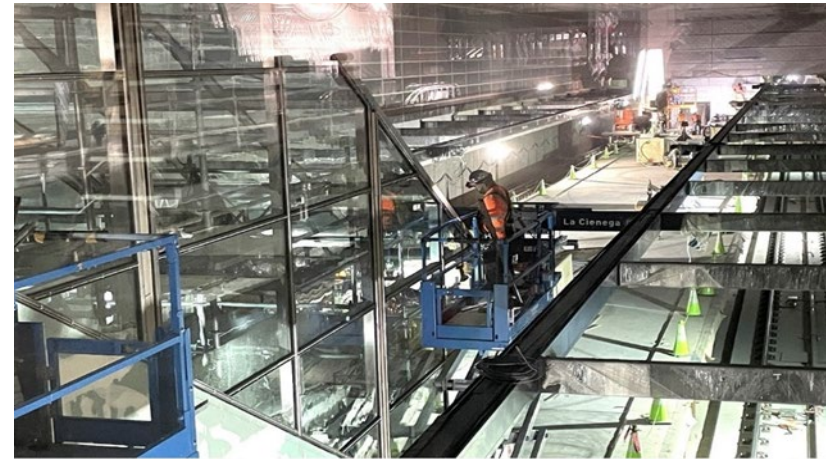
Wilshire/Fairfax Station Smoke Enclosure Glass Installation
