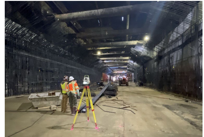
Century City Constellation Station Concourse Level Looking East
