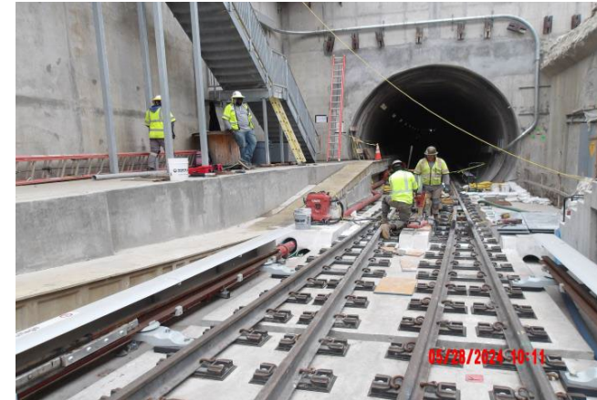
AL Portal work
