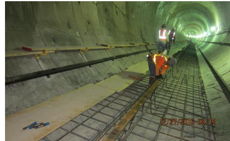
Initiating southbound tunnel concrete invert work
