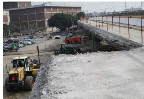
Edge of Deck Removal
