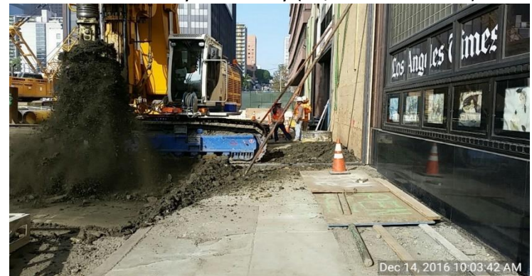
Piling on 2 nd Street (2 nd /Broadway Station)
