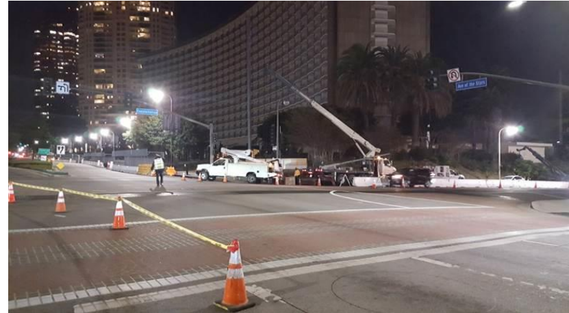
Telecom joint trench construction at Constellation Boulevard
