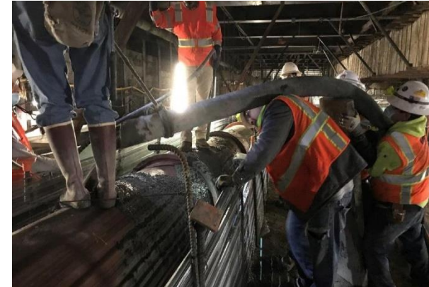
Wilshire/La Brea Concrete Placement Above Station Roof
