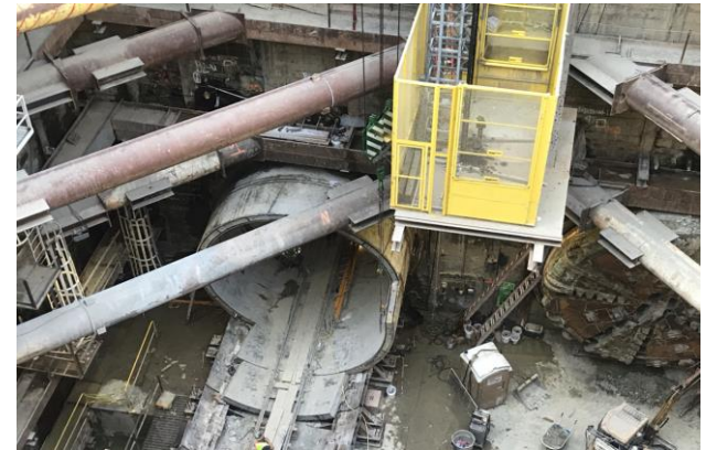
Tunnel Access Shaft
