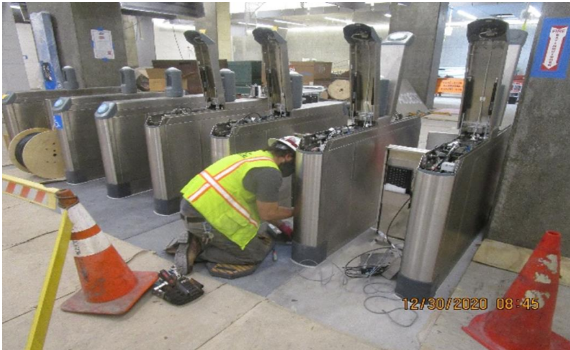
LEIMERT PARK STATION – Continue performing electrical work to the Fare Gate/TVM system at the Paid & Free Area.
