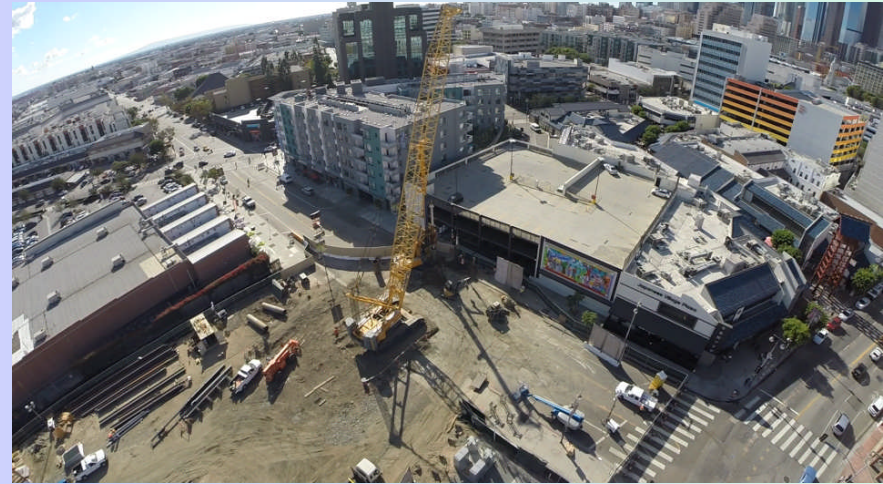
Construction Activities at 1 st /Central Station yard
