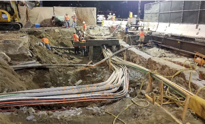
Utility work on Flower Street
