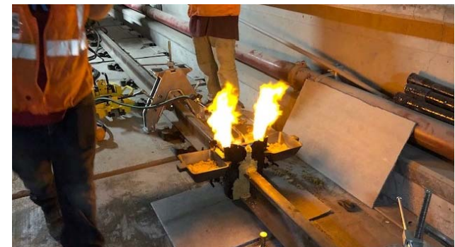
Pre-heating process for Orgo-Thermite rail welding
