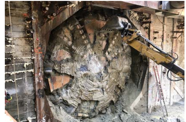
BL TBM "Ruth" at Tunnel Access Shaft
