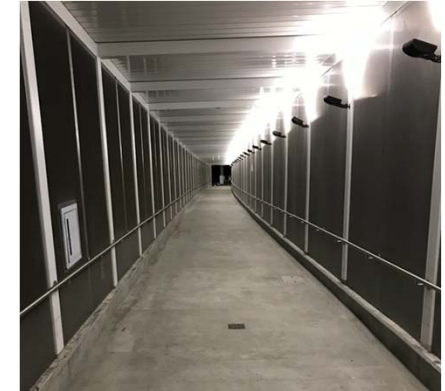
Pedestrian Ramp to Platform
