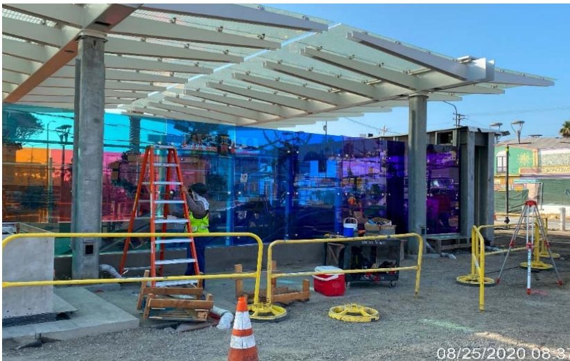
LEIMERT PARK STATION – Continue installing art glass panels around the main entrance canopy structure at the plaza level.
