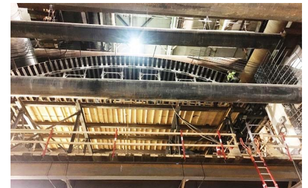
Roof Shoring Frames at Wilshire/La Cienega Station
