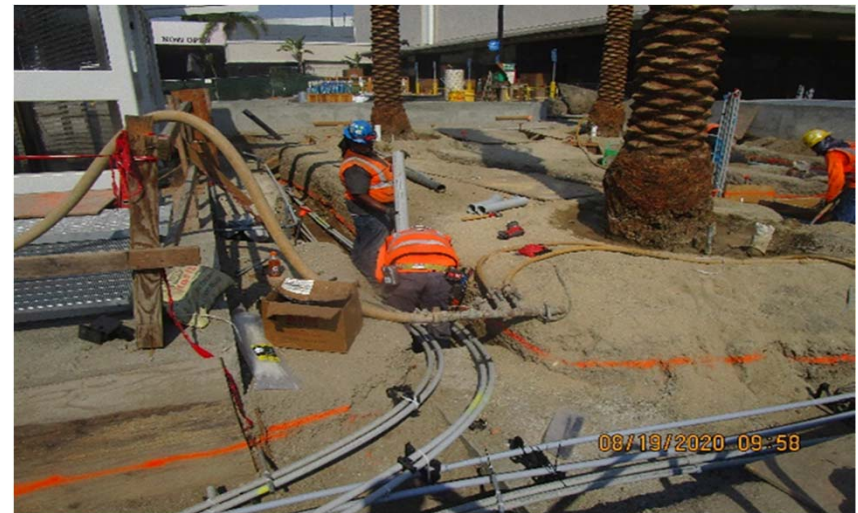
MARTIN LUTHER KING JR. STATION – Continue installing conduit for landscape lighting throughout the plaza level.
