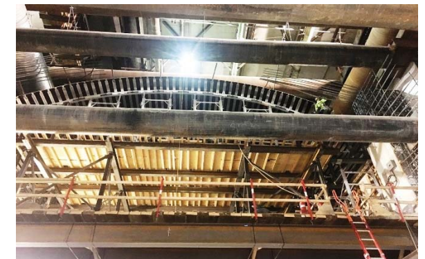
Roof Shoring Frames at Wilshire/La Cienega Station
