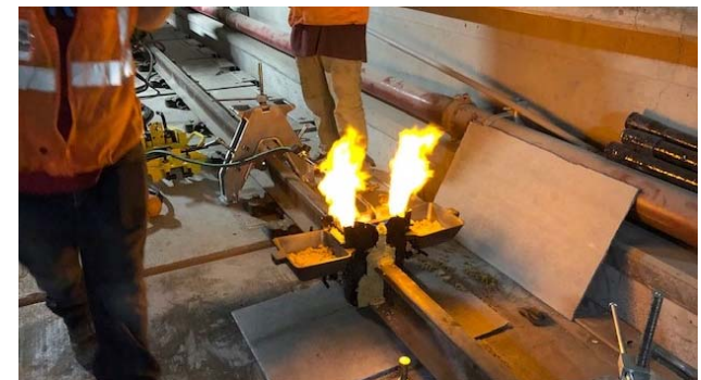
Pre-heating process for Orgo-Thermite rail welding
