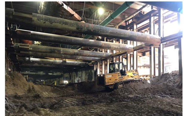
Excavation of the Wilshire/Rodeo Station
