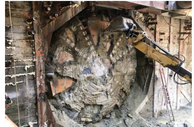
BL TBM "Ruth" at Tunnel Access Shaft
