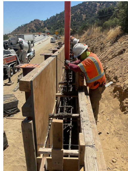
Pouring concrete at Retaining Wall 2461
