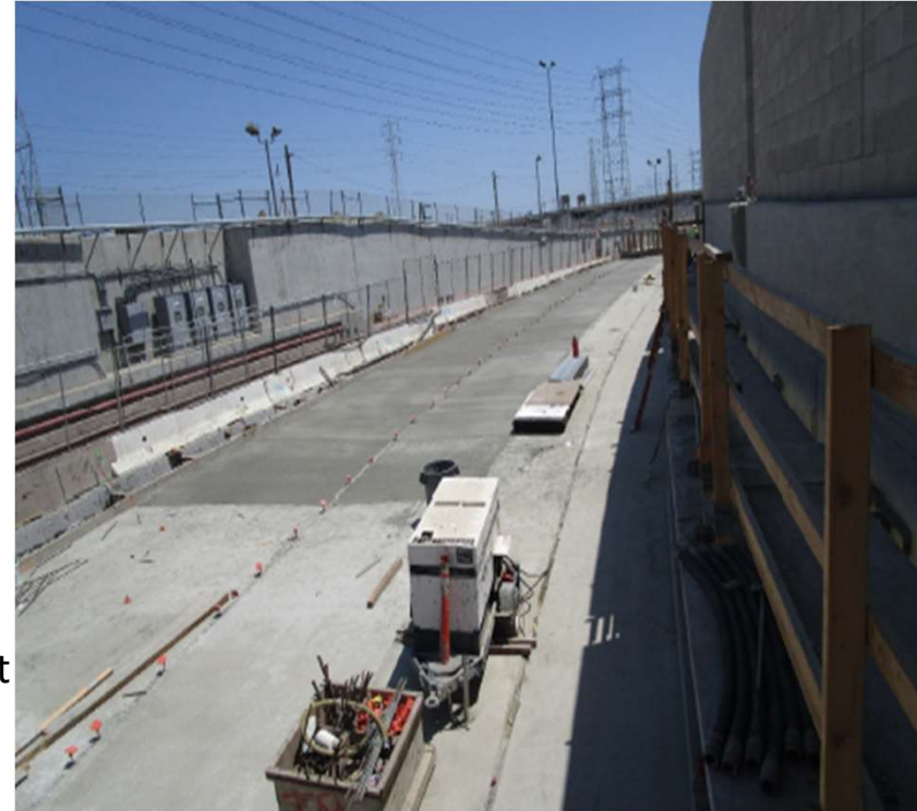
Portal –West Retaining Wall and invert
