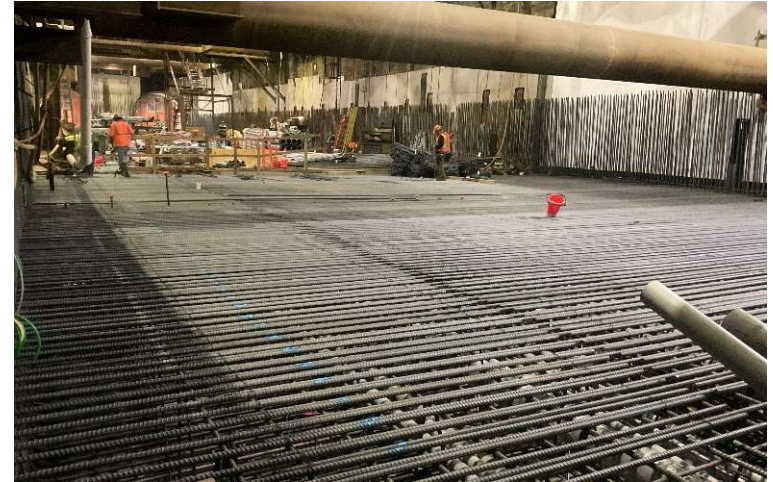
Century City Constellation Station - Top Mat Rebar
