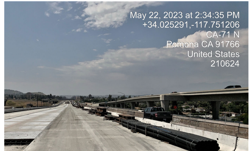
JPCP paving in the median
