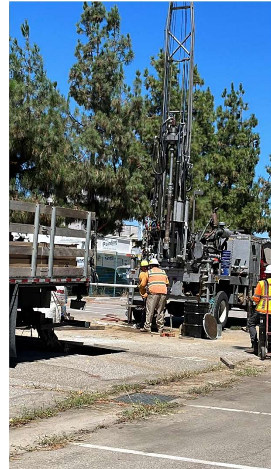
Geotech Investigations for Stormwater Capture
