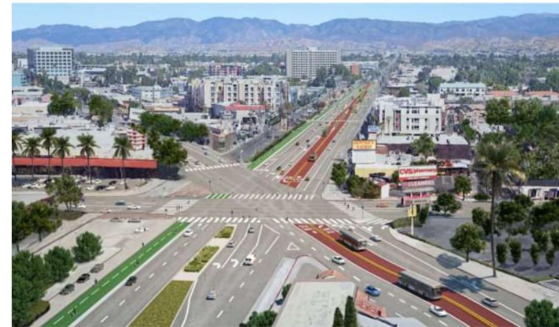
View of Vineland Ave / Lankershim Blvd
