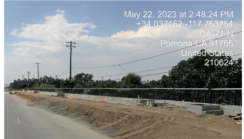
Retaining wall 161 and drainage system construction
