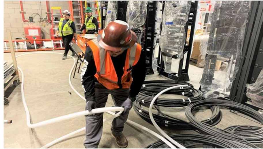
Wilshire/La Brea Communications Cable Installation
