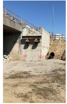
Castaic Creek Bridge Abutment 4 Complete
