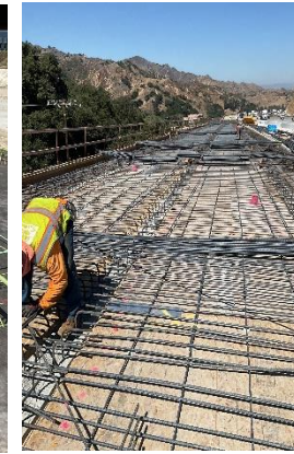
Gavin Canyon Bridge Deck Rebar Install
