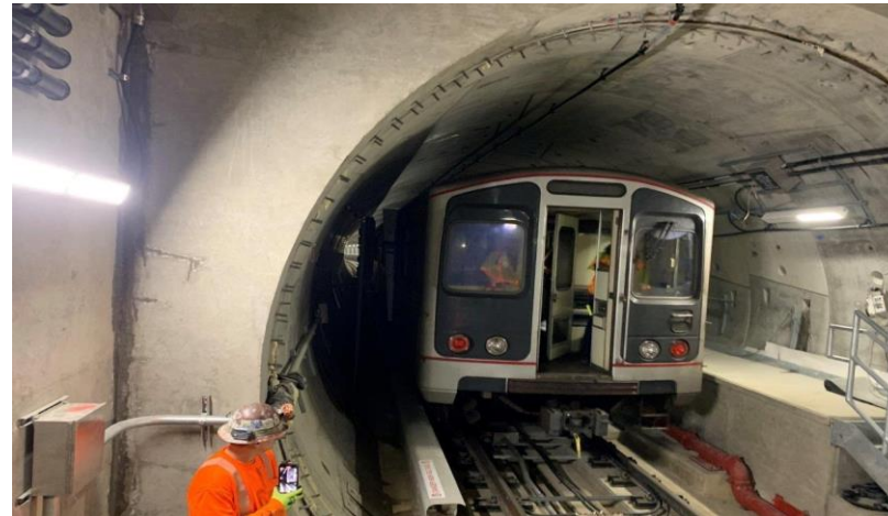
Reach 3 Tunnel (Fairfax to La Cienega) Dead Car Train Test entering La Cienega Station (BR)
