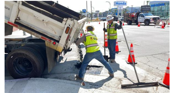
Potholing Restoration on Aetna St
