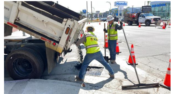
Potholing Restoration on Aetna St
