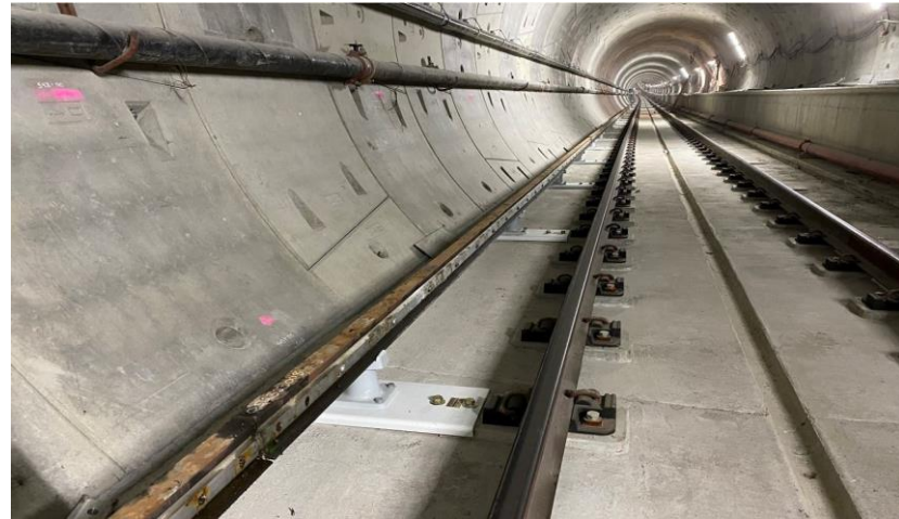
Reach 3 Tunnel (Fairfax to La Cienega) Contact Rail Installation
