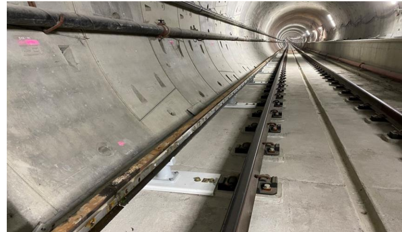
Reach 3 Tunnel (Fairfax to La Cienega)
