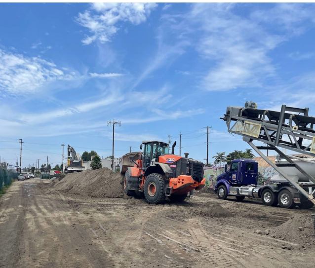
Processing Hazardous Soil
