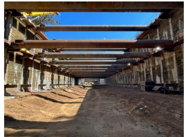
Westwood/VA Station: Excavation Level 3 Support
