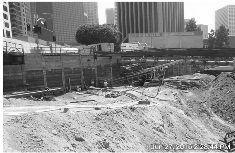
Structural excavation at 2 nd /Hope
