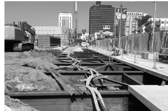
Wilshire/La Brea Station South Deck Beams
