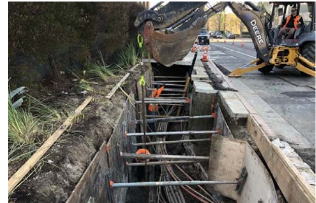
AT&T Utility Work in Century City
