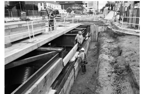
Decking Operation at Wilshire/Fairfax Station
