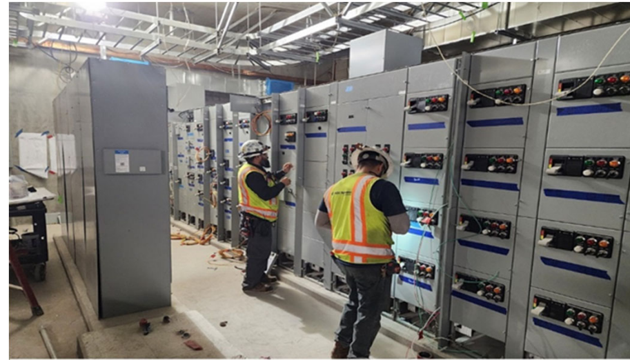
Wilshire/Fairfax Testing Motor Control Center
