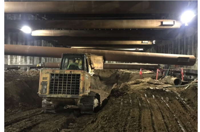
Westwood/UCLA Station: Placement of BL3 Strut
