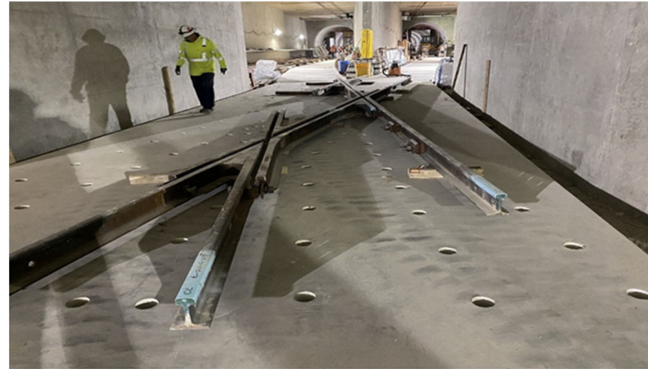
Reach 3 Tunnel (Fairfax to La Cienega) Placement of Diamond Grid Rail
