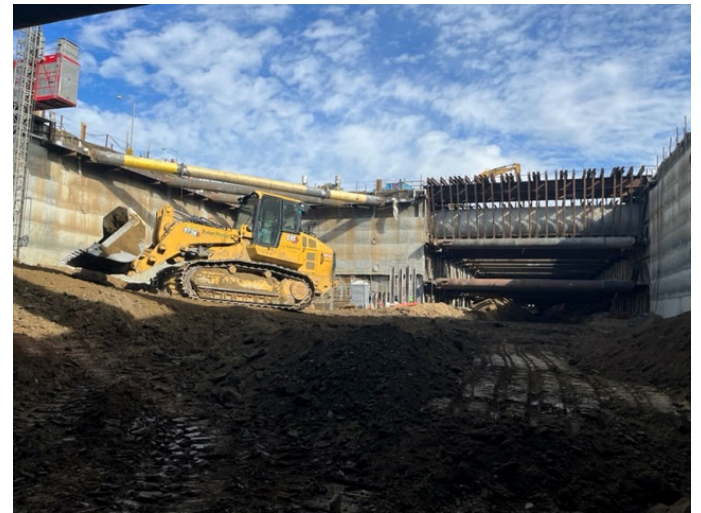
Westwood/VA Hospital Station: Excavation for Level 4 Support
