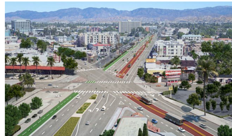
View of Vineland Ave / Lankershim Blvd
