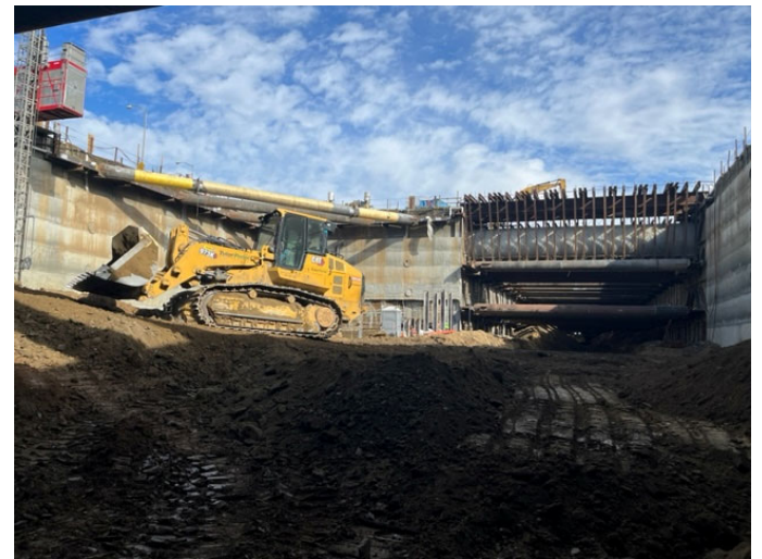
Westwood/VA Hospital Station: Excavation for Level 4 Support
