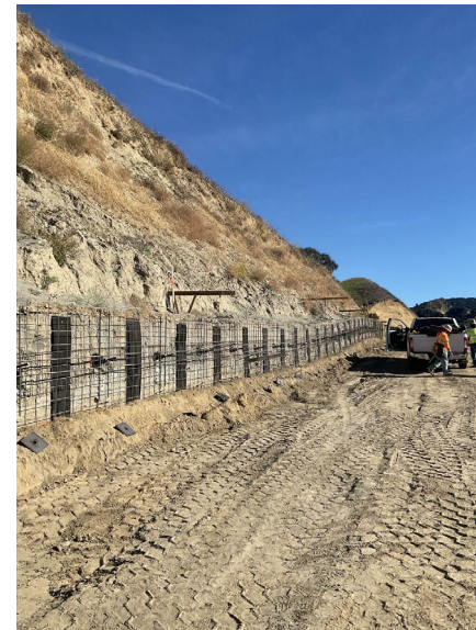
Soil nail installation at Retaining Wall 2524
