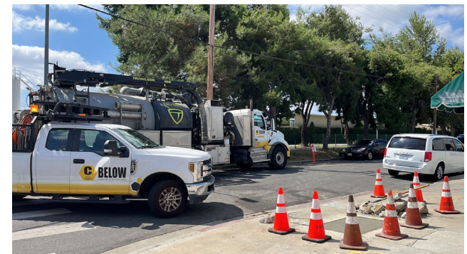
Sidewalk Panel Restoration on Bessemer St
