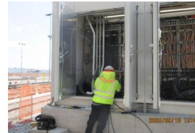
Train control cable installation at Bungalow B
