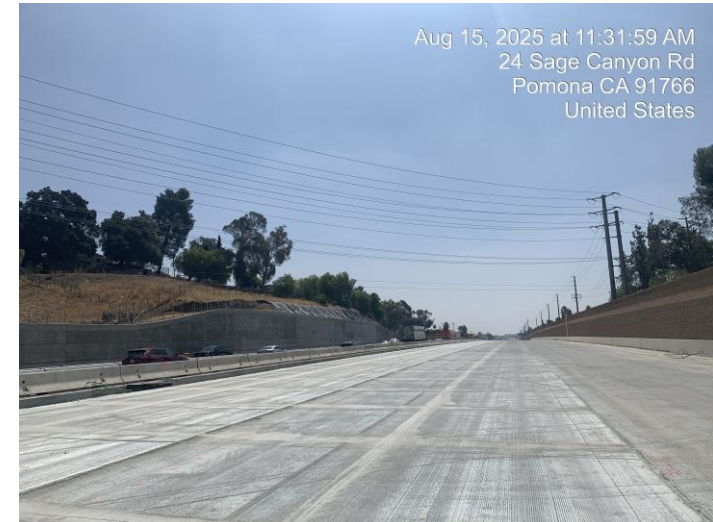
Stage 3, SB-71 paving.
