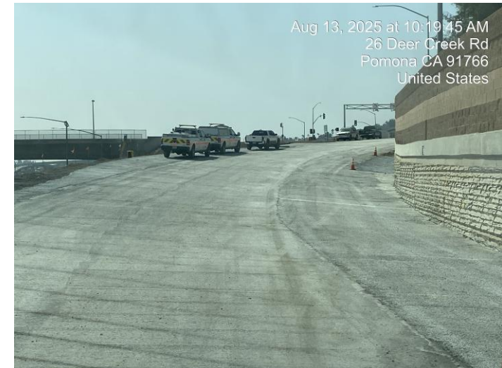
Realigned SB Rio Rancho off-ramp, LCB paving.
