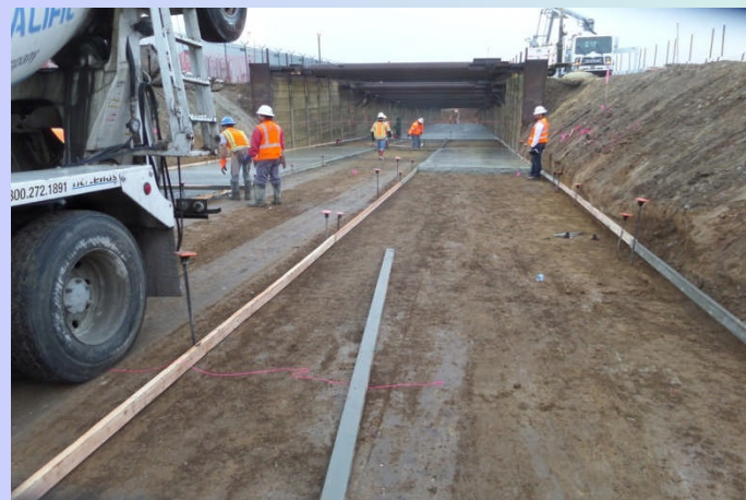
Placement of mud slab at UG#1 (near LAX runways).
